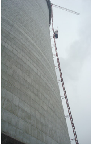
山东济宁电厂冷却塔用SC120曲线施工升降机 SCQ120 Curved Hoist for cooling tower of power plant, Shandong
