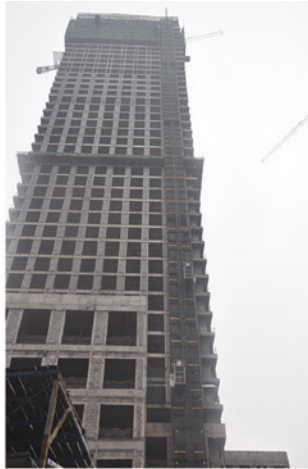
天津渤海银行240米变频调速升降机 Tianjin Bohai Bank Mansion, VVVF building hoist (240m)
