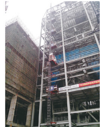
安徽合肥电厂SC200/200变频施工升降机 SC200/200 (VVVF) for Hefei Power Plant of Anhui province
