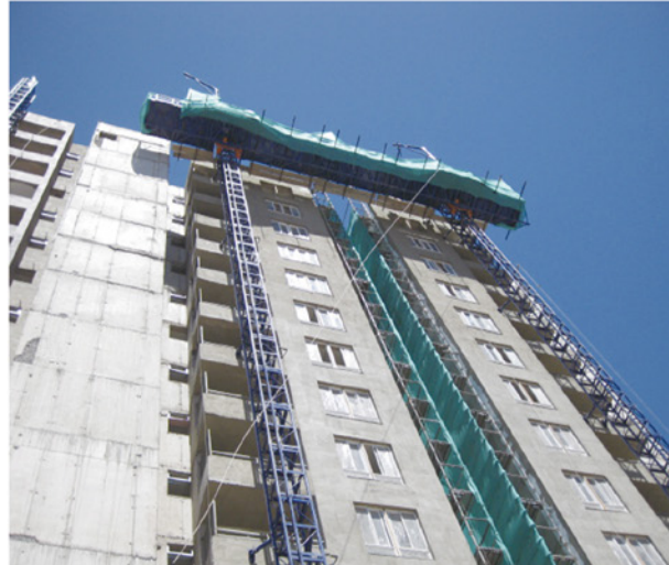
智利施工平台 Chile, working platform
