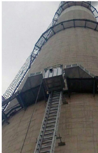
梅县荷树园电厂SC50工业电梯 SC50 Industrial Hoist for Heshuyuan Power Plant in Mei County
