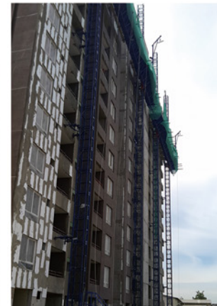
朝鲜柳京大厦SCP400施工平台 SCP400 for Liu Jing Building, North Korea
