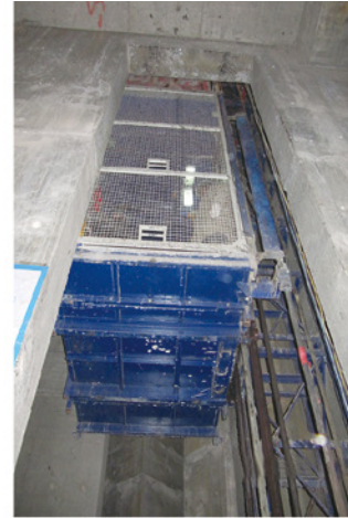
宁夏巨元万象大厦263米井道施工升降机 Ningxia Genyuan Building, Installed in Elevator Shaft (263m)
